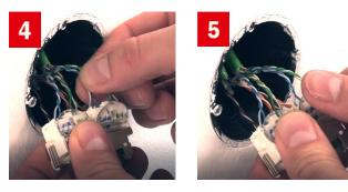
Insert wire pairs into the holes of the sliders to the stop according to the printed color code. Visually check before closing. Then close the lever by pressing it down with your finger.
