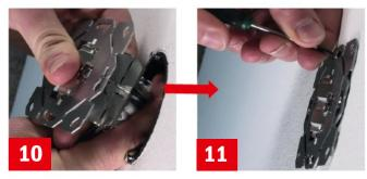
Press the module with the mounting plate into the wall box and make sure that none of the wires are squeezed. It is recommended to give the wire pairs a slight S-shaped bend (see Figure 10). Screw the mounting plate firmly in place.
