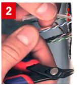
Set down the cable sheath 60 mm and cut off the inner plastic strand and the thread.
