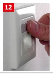
Install central cover and (optional) cover frame by fastening the pre-assembled screw and insert labeling strip or printed label (up to 10 mm width).
