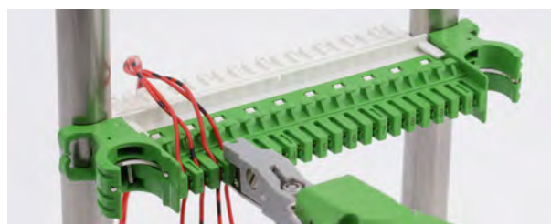
Connecting the cable side
